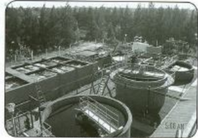
Aerial view of treatment plant
